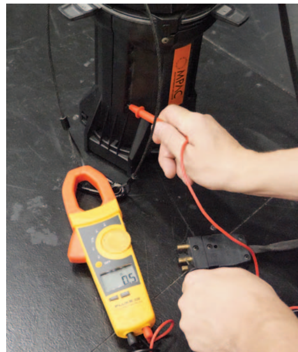
A multimeter can check the ground continuity between the connector and the equipment's housing.
