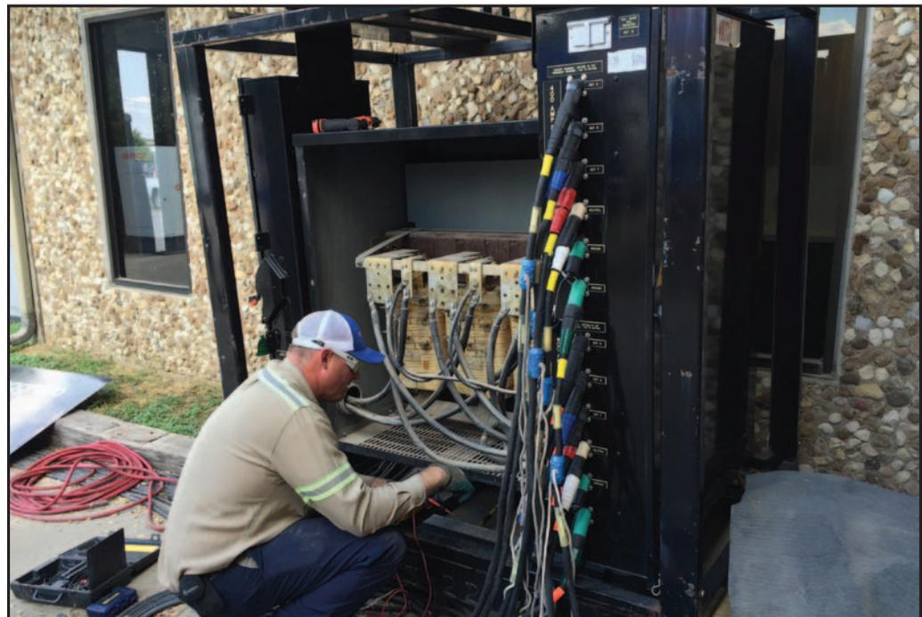
Figure 1 – A transformer that hums loudly and produces a lot of heat with no load connected to it is very likely failing. This power tech attempted a diagnosis after de-energizing the generator and transformer.
