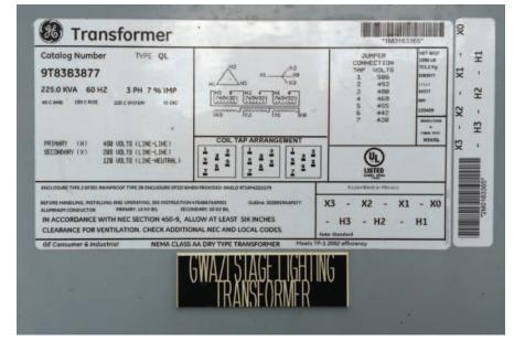
Figure 3 – The nameplate on a feeder transformer provides a lot of useful information about the operating conditions of the device including the kVA, frequency, primary and secondary voltages, impedance, clearance, class of insulation, ambient temperature rating, rise temperature, and more.
