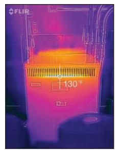
Figure 5 – An infrared camera can uncover hot spots in electrical apparatus that could indicate pending failure. If the equipment can't be de-energized for an IF scan, you can still get clues about the health of the apparatus.
